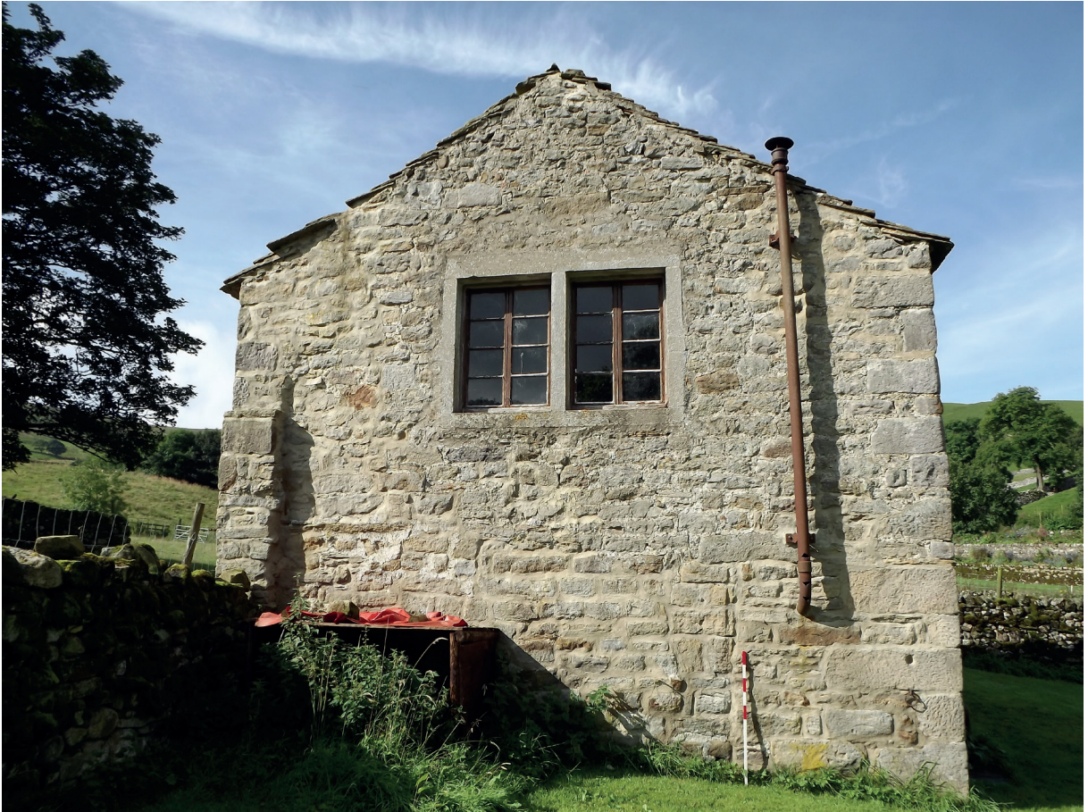
Figure 8 Mitchell House, Thorpe, view of northern gable end.
