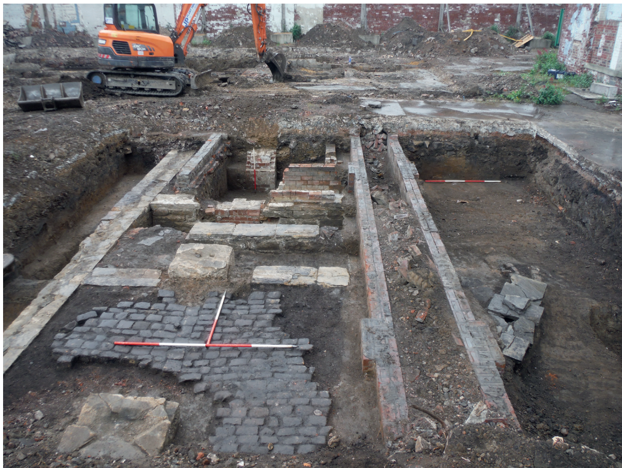
Figure 7 Globe Foundry Foundations.
