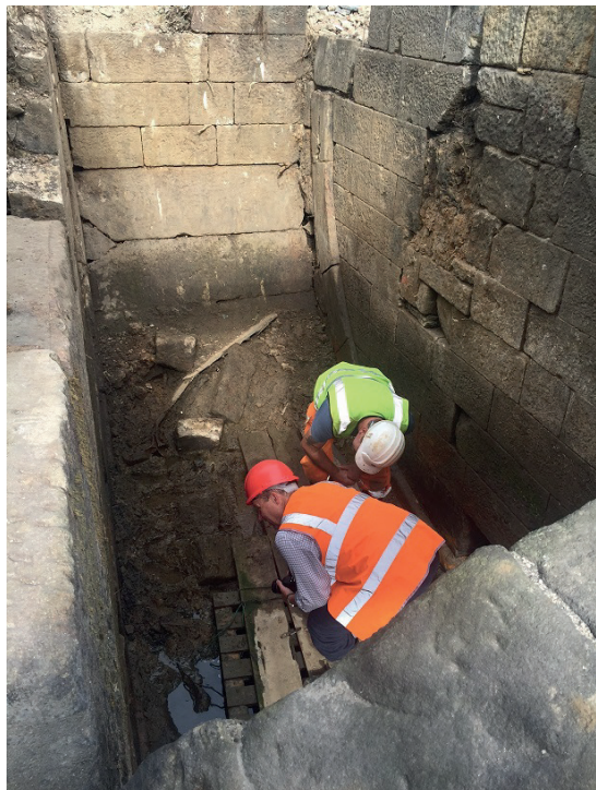
Figure 10 Water wheel pit.
